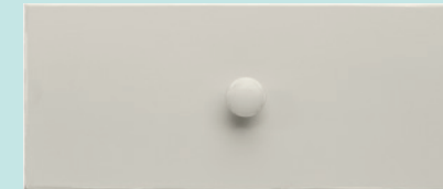
WEATHERED PAINT FINISH
